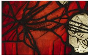
The damage in this area of the window was most likely caused by the impact of a thrown stone (or a similar object) as the breaks in the glass radiate from a central point. The only way that restorers in the past were able to repair such damage was
