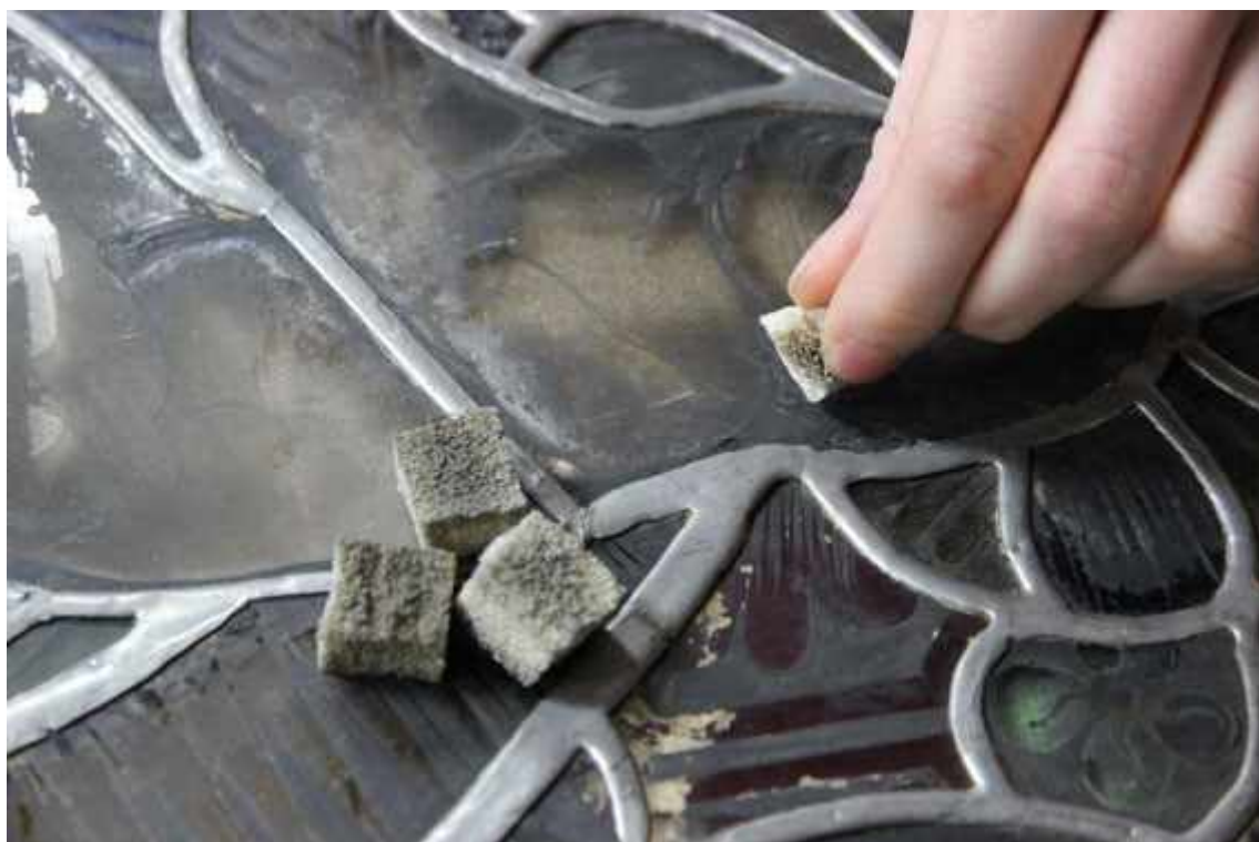
REMOVING LOOSE PARTICLE DIRT WITH SMOKE SPONGES.
