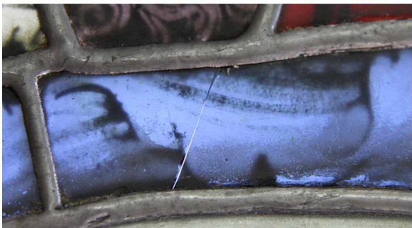
Fracture before polyester is applied (transmitted light)
