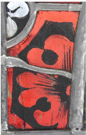
Fracture after polyester has been applied (front transmitted light)
