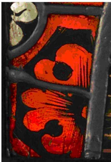
Fracture before polyester is applied (front transmitted light)
