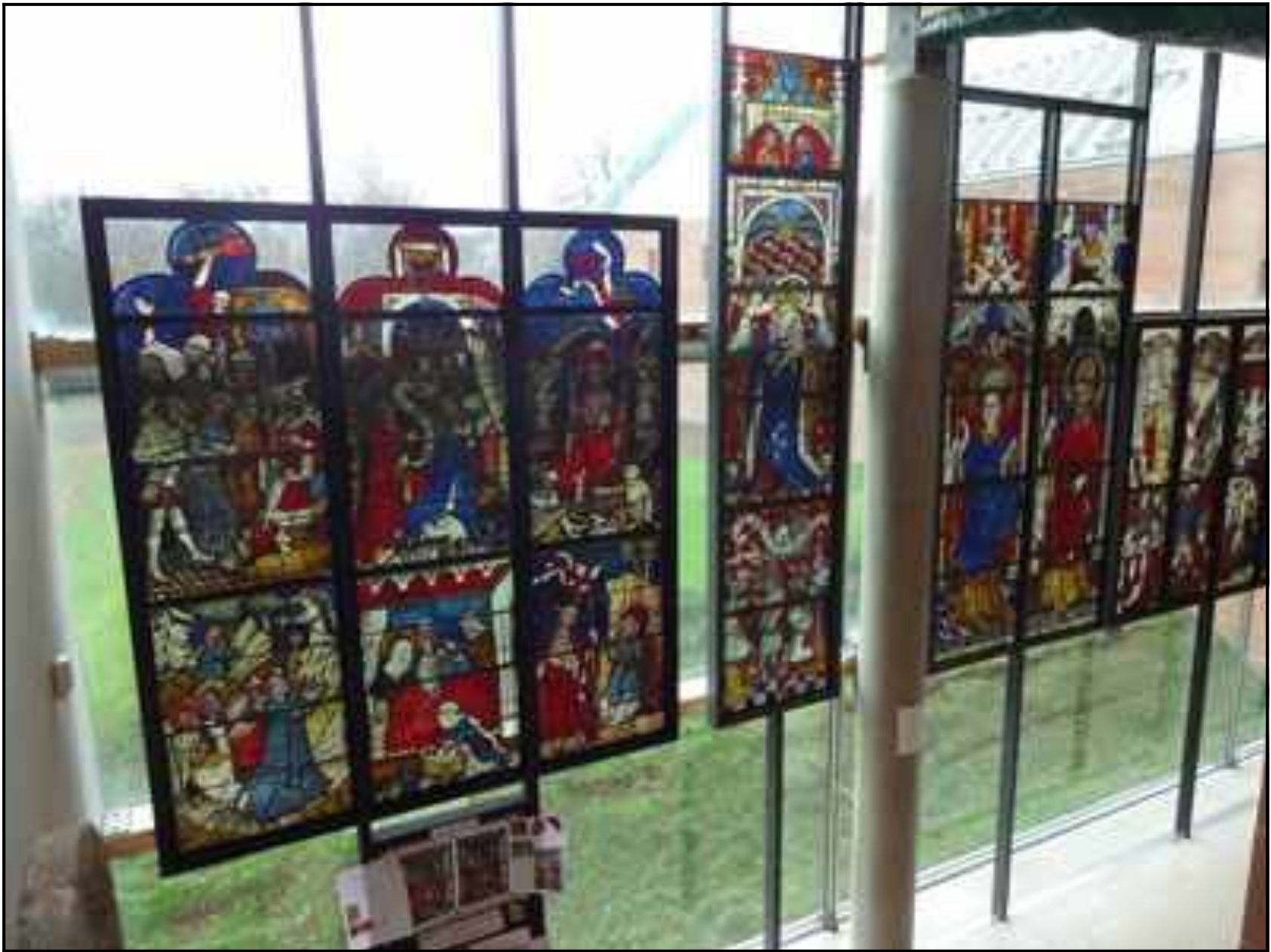
The completed reinstallation including the two Bishop Saints. The small top panels have been omitted as they are close to the high humidity in the ceiling.
